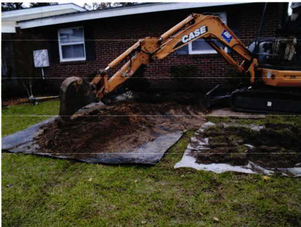
Picture 2: UST 555Dahlia excavation in progress.
